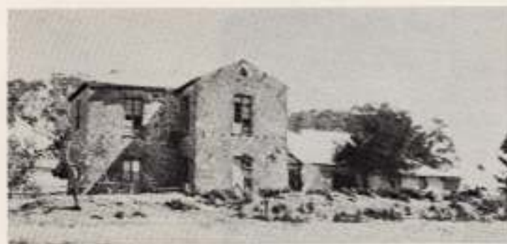
"The Vallies" — a ruined Homestead.
